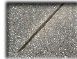
Floor Cutting : 8 x 12mm
